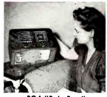
**RCA** "Roto-Base" ★ Little Nipper model 46X23, with new RCA "Roto Base" feature, which acts like a turntable for entire set, obtaining maximum signal strength from Magic loop antenna. and greater tuning ease. RCA Mfg. Co., Camden, N. J.—RADIO TODAY.
